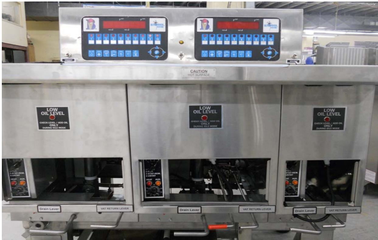
The 14" vat has two 8.5 KW elements for at total 17KW wired for 3 phase power. At 208 volts the amp load/vat is 47 amps. The shortening capacity for the high level is 45lbs, while the low level is 35 lbs. Each vat has an individual selector control box for operating the vat. (see page 7 for instructions).
